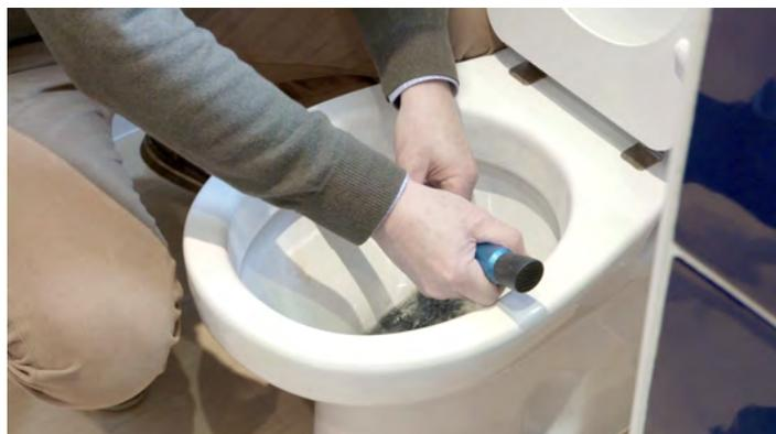
Stand at the side of toilet holding the wider tube with the longer narrow tube pointing towards you, carefully place the black end of the narrow tube under the rim of the pan closest to you, ensuring that the angled end fits securely under the rim. Pull back on the wider tube and slide the other end of the bar under the rim on the other side. The springs will adjust to your toilet's pan width and hold the bar in position.
