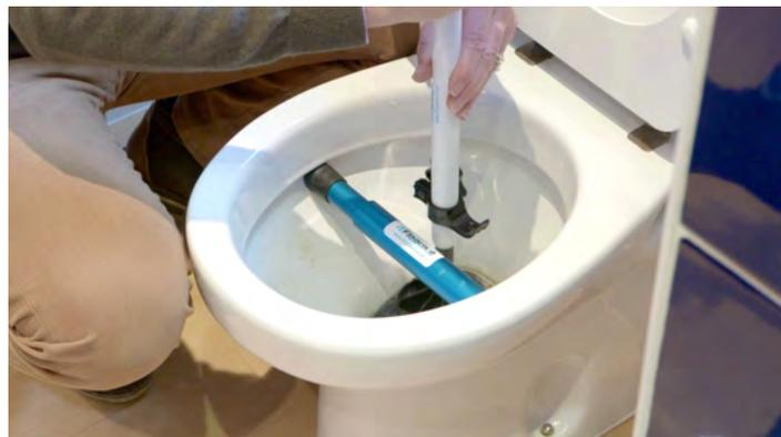
Place the white FloodKit® Toilet Strut so that the plunger head is close to the centre of the bag, just behind the Blue cross bar with the hand wheel facing the cistern. Push down on the strut and turn 90 degrees clockwise so that the lug locks into position under the cross bar
