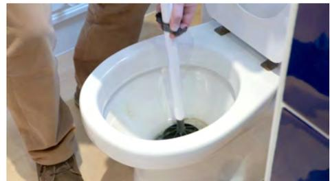
Place the bag into the throat of the U Bend, and use the white Strut with the plunger at the end to push firmly into place.
